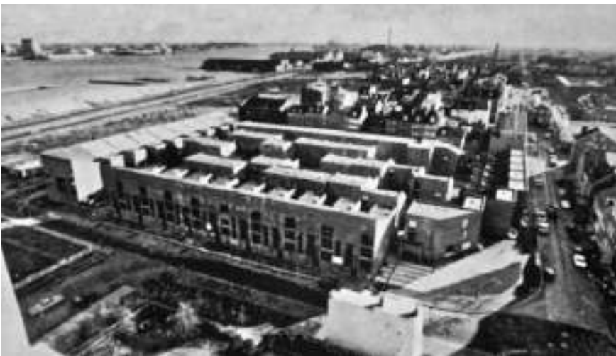
Fig. 116. View from the Delaware River towards Front Street.
